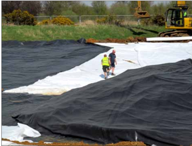
New lining being installed 24th April 2013
